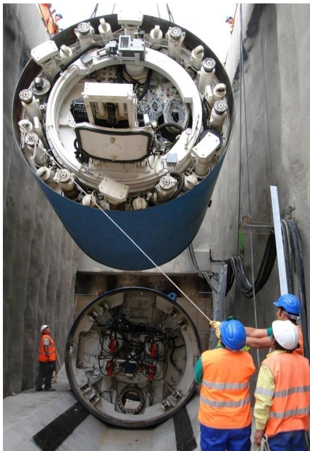
EPB TBM assembly
