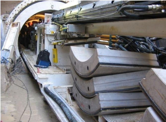
Segmental linings in the TBM back up.
