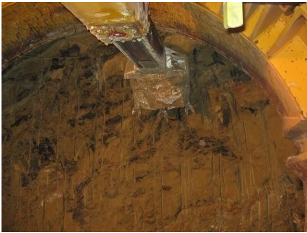
Open shield excavation face with excavator
