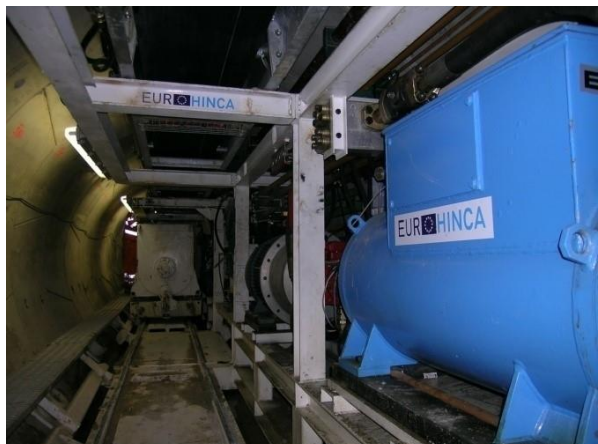
EPB TBM Back up inside the tunnel
