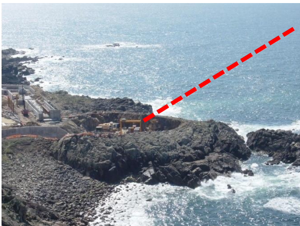
Submarine outfall launching shaft. A corula
