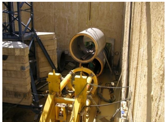
Laying of a section of pipe for jacking.
