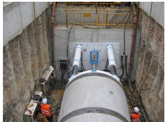
Launching shaft with thrust system.
