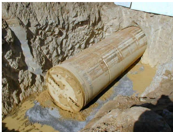
TBM exit in reception shaft.
