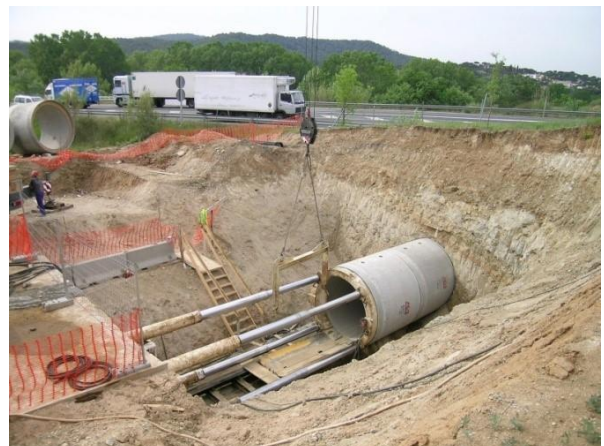
TBM crossing under road.
