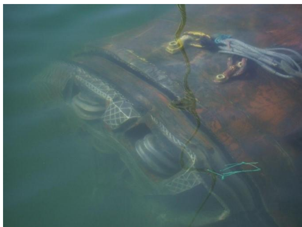
TBM rescue after underwater outfall.
